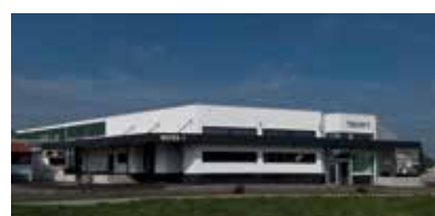
factory for elements, Ried i. I. Upper Austria
